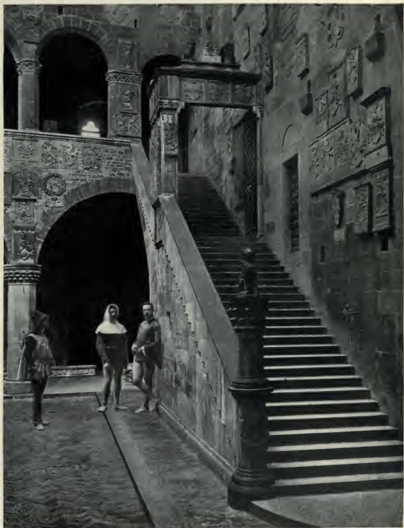
THE BARGELLO (PALACE OF THE PODESTÀ)—STAIRS OF HONOUR
